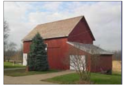
Daniel Garfield Barn at 5013 Detroit Road before it was taken down in 2005.
